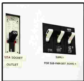
Main Breaker: 125 amp / 3 phase
